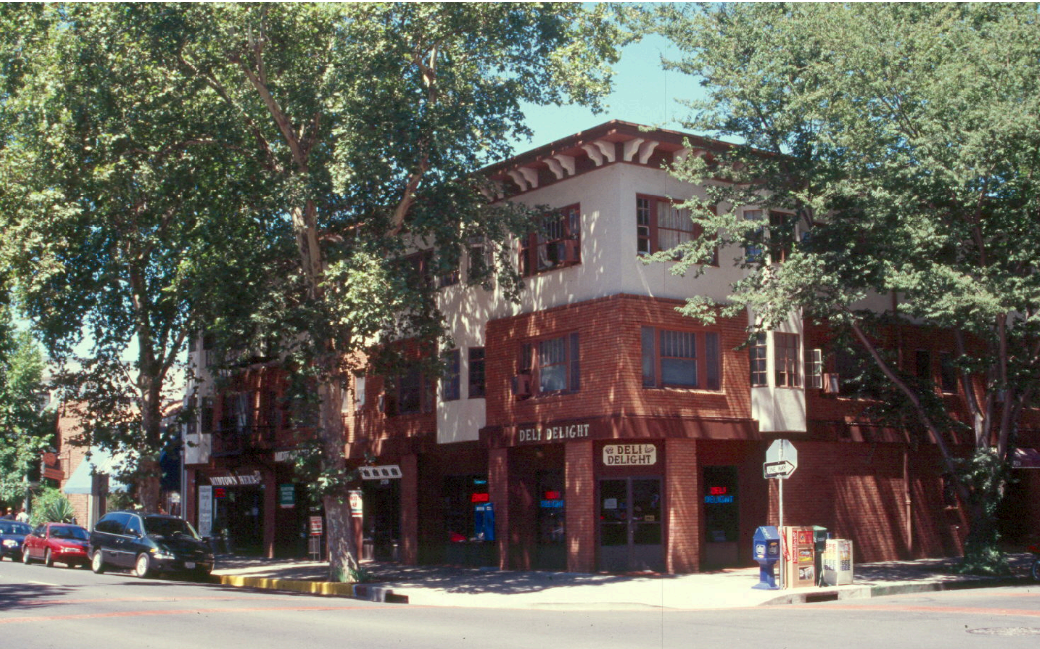
Housing over retail shops
